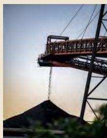
Front cover: Ernest Henry Operations - sunrise at conveyor 5
